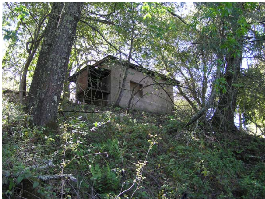
Image 70. Alma College CMU Shed, existing exterior view from the south. The shed is constructed of concrete masonry units and did not appear historic. (Knapp Architects, digital photograph, 2009)
