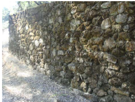
Item 19 090701 Stone retaining wall
