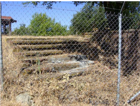
Item 14 090701 Brick stair from
