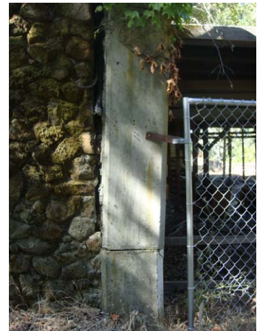
Item 19 090701 Stone retaining wall
