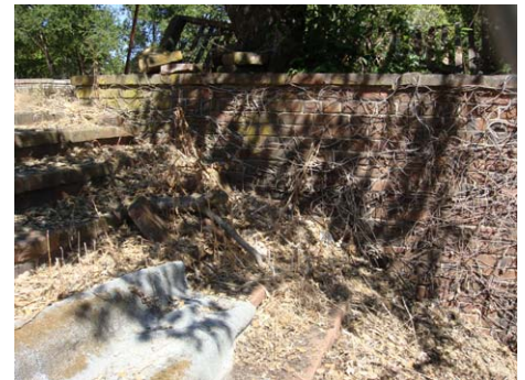
Item 14 090701 Brick stair from
