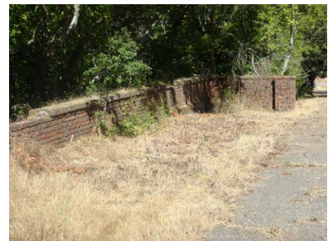
Item 21 090701 Brick retaining wall SE
