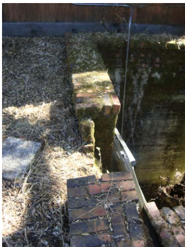
Item 20 090701 Brick retaining wall on
