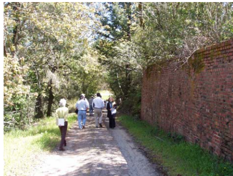
Item 23 Brick retaining wall at site
