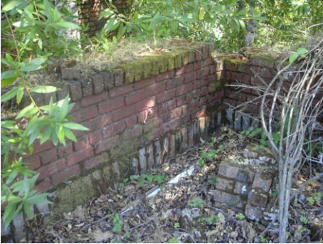
Item 18 090701 Brick retaining wall
