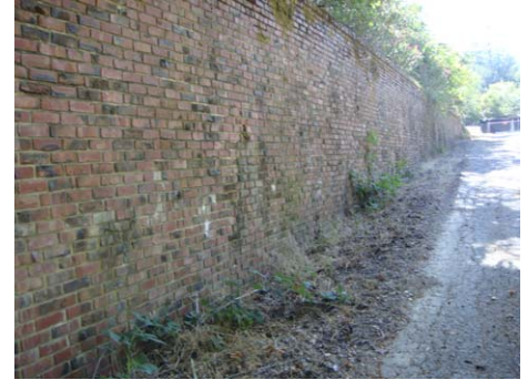
Item 23 090701 Brick retaining wall
