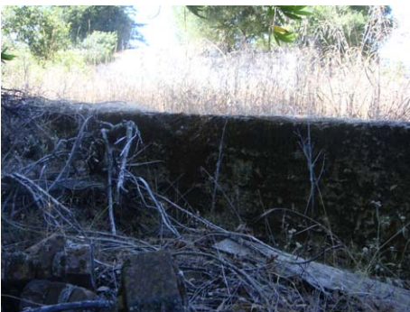
Item 18 090701 Brick retaining wall
