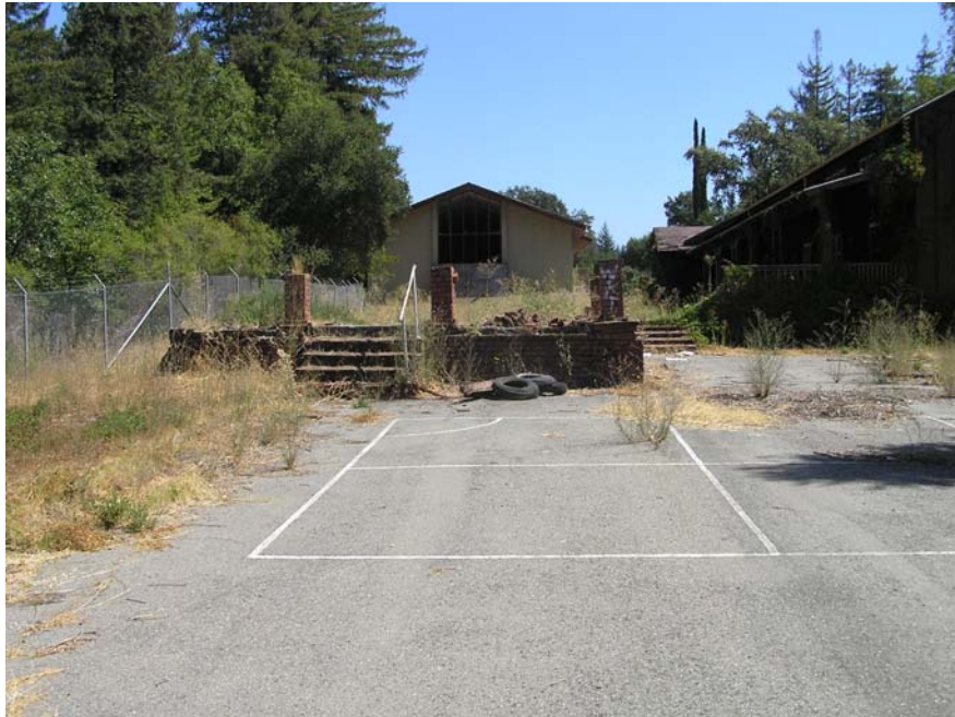
Image 57. Alma College Dormitory porch ruin, exterior view looking east toward 1949 Library. The brick porch ruin connected the dormitory (left) and classroom (right). The brick paving, stairs and a few piers remain. (Knapp Architects, digital photograph, 2009)
