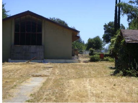
Item 27 090701 Ped circulation near
