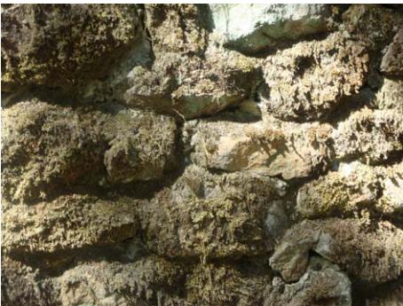
Item 19 090701 Stone retaining wall
