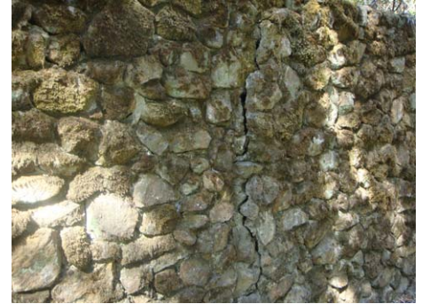
Item 19 090701 Stone retaining wall
