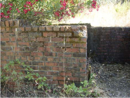
Item 23 090701 Brick retaining wall
