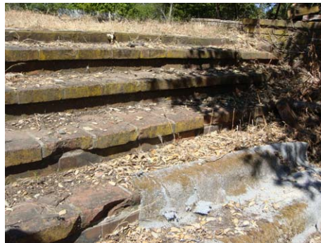
Item 14 090701 Brick stair from
