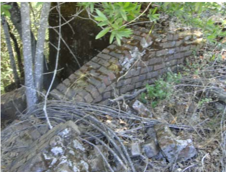
Item 18 090701 Brick retaining wall
