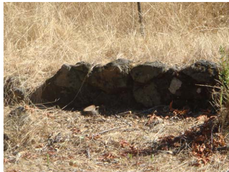
Item 22 090701 Rock retaining
