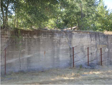
Item 15 090701 Concrete retaining
