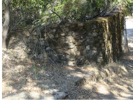
Item 19 090701 Stone retaining wall
