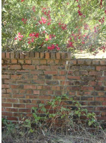
Item 23 090701 Brick retaining wall
