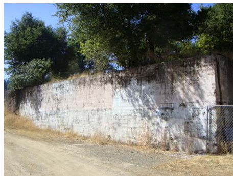
Item 15 090701 Concrete retaining
