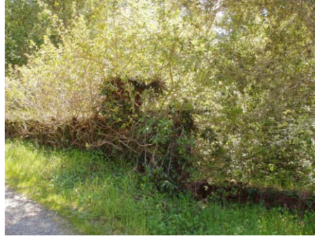
Item 12 0904xx Brick retaining wall
