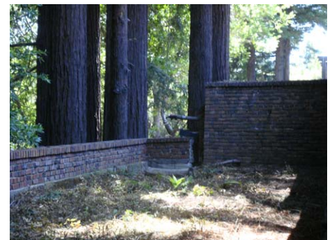
Item 27 090701 Ped circulation near
