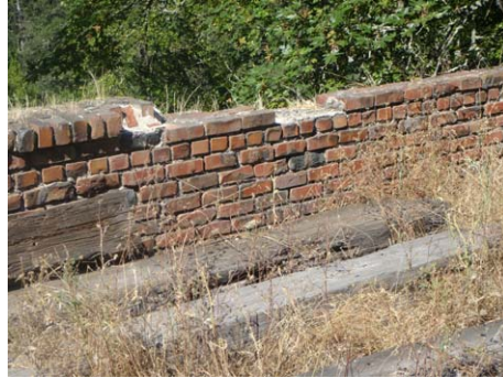
Item 21 090701 Brick retaining wall SE
