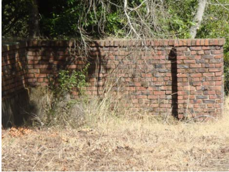
Item 21 090701 Brick retaining wall SE
