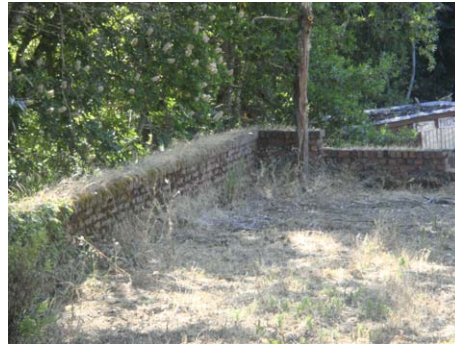
Item 26 090701 Brick retaining wall
