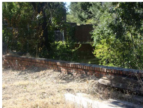
Item 21 090701 Brick retaining wall SE
