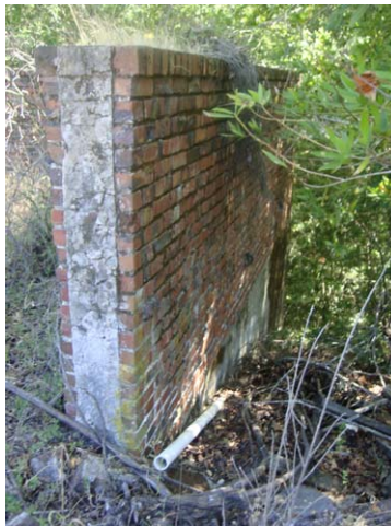
Item 18 090701 Brick retaining wall
