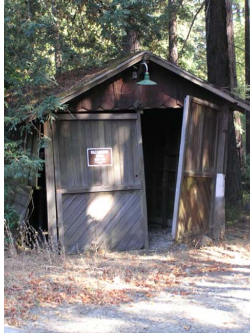
Image 67. Alma College Wood Shed, existing exterior view of west façade with decorative wood shingles and framed barn-like doors. (Knapp Architects, digital photograph, 2009)
