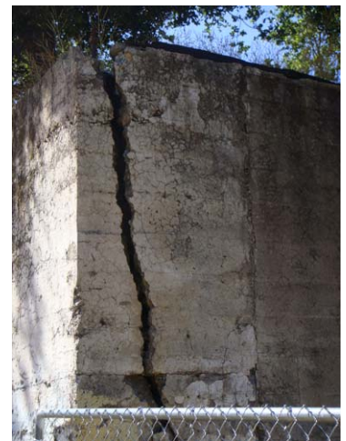
Item 15 090701 Concrete retaining
